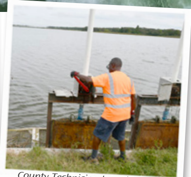
County Technician lowering flood control at Lake Seminole.
